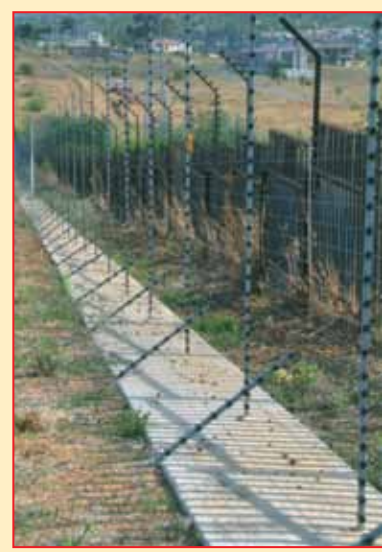
Existing anti-dig methods, while they can be effective, are expensive and time-consuming to install.
